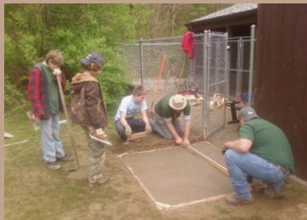
kennels, clearing a couple of drainage pipes, and pouring a 4'x5' concrete pad — a first-time activity for most of the boys. In the picture at left, Messrs. Peschock and Gillham give the boys some tips on floating.
