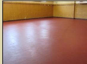
In addition to the gym floor, shown here with just the first coat of paint, Steve and crew tackled the floor of the anteroom, using the paint that was left over from the first coat. The door to the dining room, which had scraped the floor through most of its arc, was realigned so as not to ruin the new paint.
